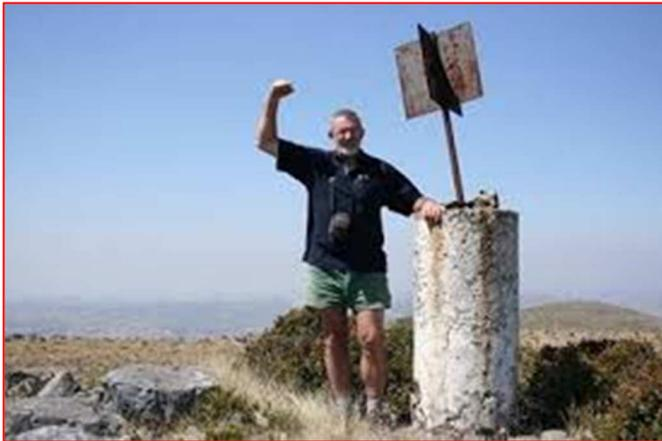
This trig beacon is in dire need of maintenance. The pillar requires some concrete and a new coat of paint. The rusty vane needs to be replaced and repainted as well
